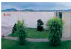
The New Factory
